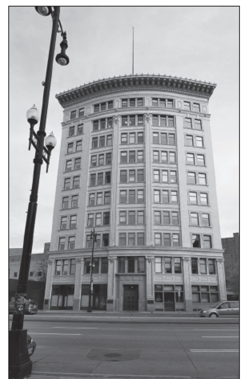
Our first home, the Confederation Life Building, 457 Main
